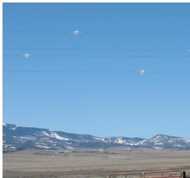
Plate 1: Electricity line marked with swan flight diverters
